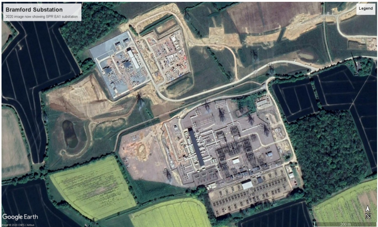
Figure 3 – As built GIS extension to NGET substation at Bramford
